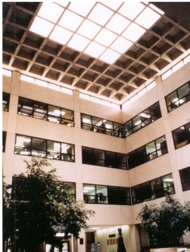
Figure 8.31 Photo of Interior View of Kleberg Animal and Food Science Center, Texas A&M University, College Station, TX
